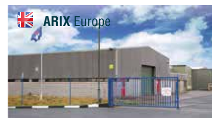
ARIX Europe Unità Logistico-Commerciale UK, Irlanda e Nord Europa Northern Europe Sales and UK & Eire Distribution Total Area: 48.500 mq - Buildings: 3.000 mq
